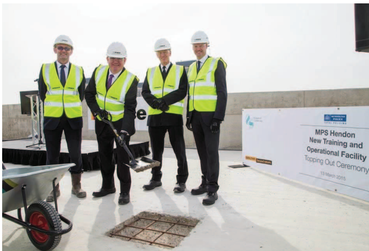
Deputy Mayor for Policing and Crime Stephen Greenhalgh and Commissioner Bernard Hogan-Howe at the topping out of the new Hendon Training and Operational Facility
